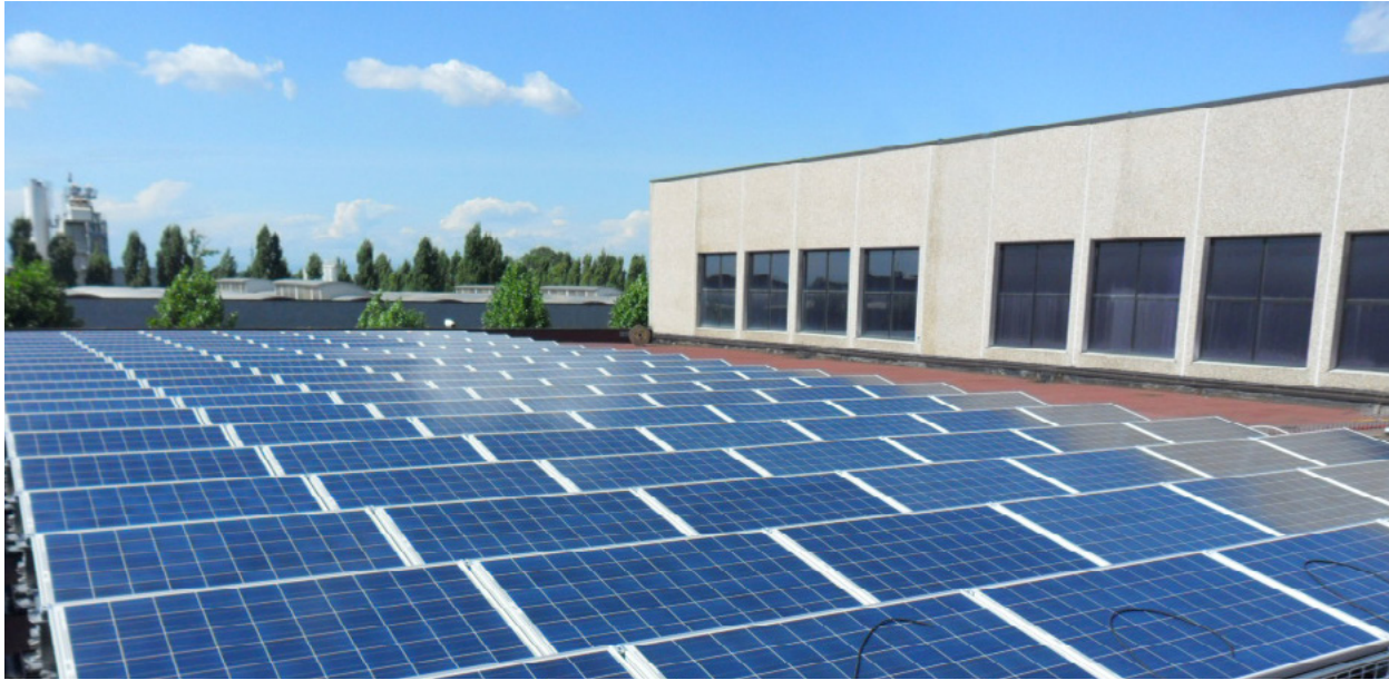
On our warehouse in Carpiano, Italy, we have installed solar panels with a yield of 250 MWh. We are growing the number of photovoltaic systems installed on our buildings worldwide.
